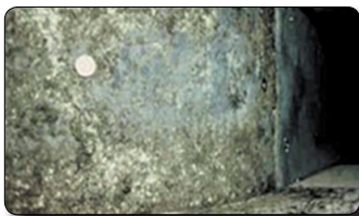
Result w/ Fibrous: Mold growth on insulation
