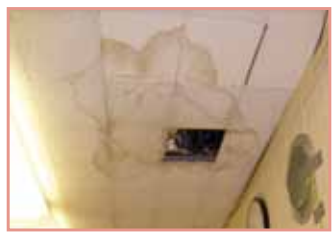
Result w/ Fibrous: Mold growth on ceiling from water drip or corrosion of duct
